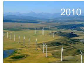
123 MW Ardenville / Kent Hills 2
